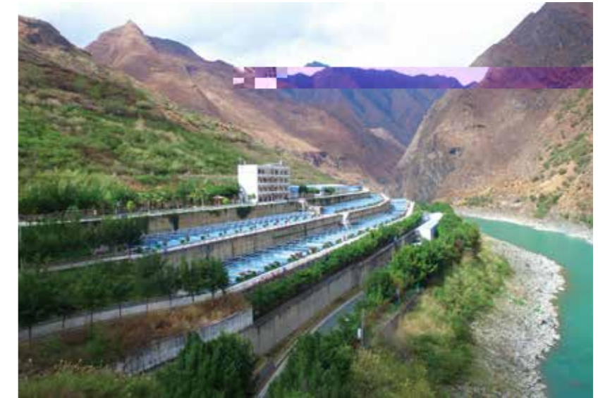
Yalong River Jinping-Guandi Fish Breeding and Release Station
