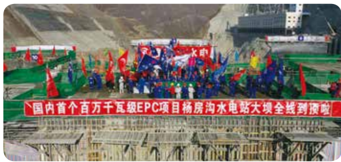
Concrete pouring completed in construction of Yangfanggou hydropower station along the Yalong River
