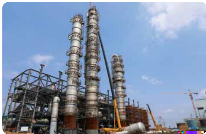
Main facility of SDIC Bioenergy Hailun Co.'s fuel ethanol project with an annual output of 300,000 tons, which now is under construction
